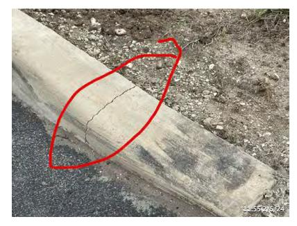
Lanier Road. Assigned To EPG. The East side parking lot entrance curbing is cracked.
